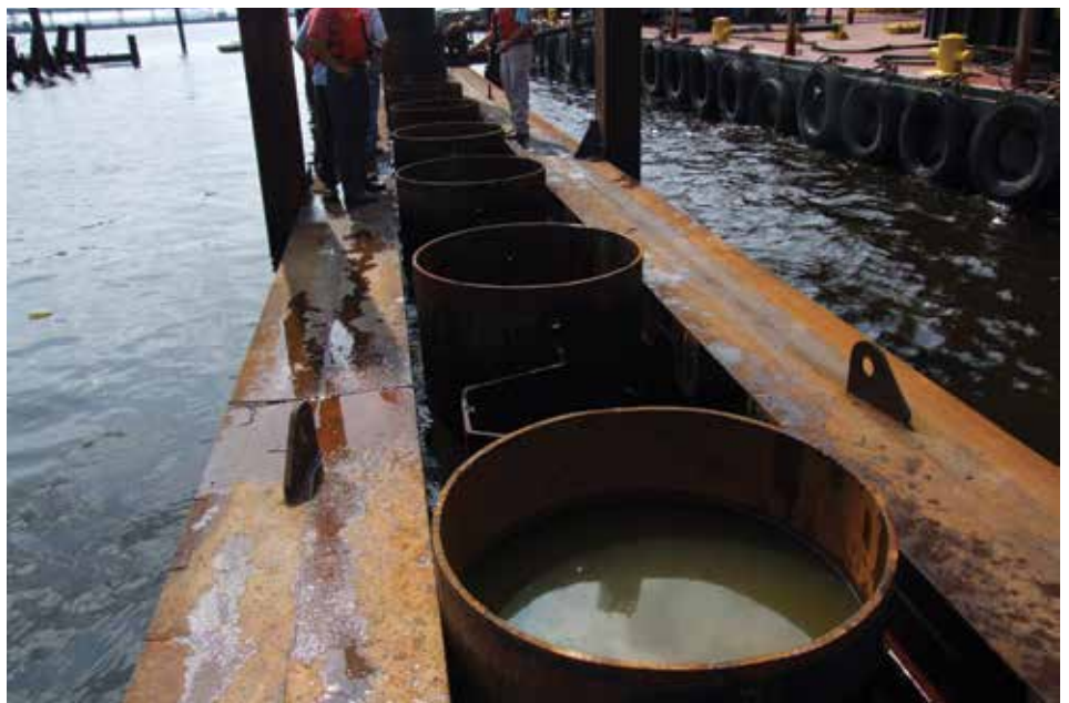
Pipe-AZ Installation Template
