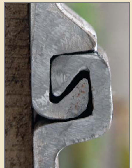
The Larssen four-point connection on AZ sheet pile is the tightest interlock design available today
