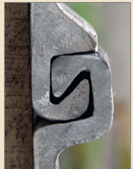
Larsen interlock connection
