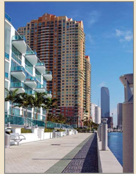
Waterfront and coastal properties are a popular draw, but come with difficult construction issues
