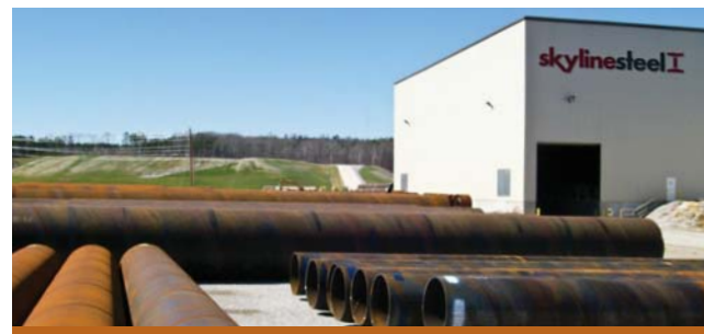
Flagship pipe facility in Iuka, MS
