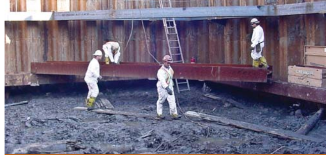
Sheet pile for environmental remediation
