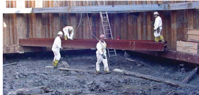
Sheet pile for environmental remediation
