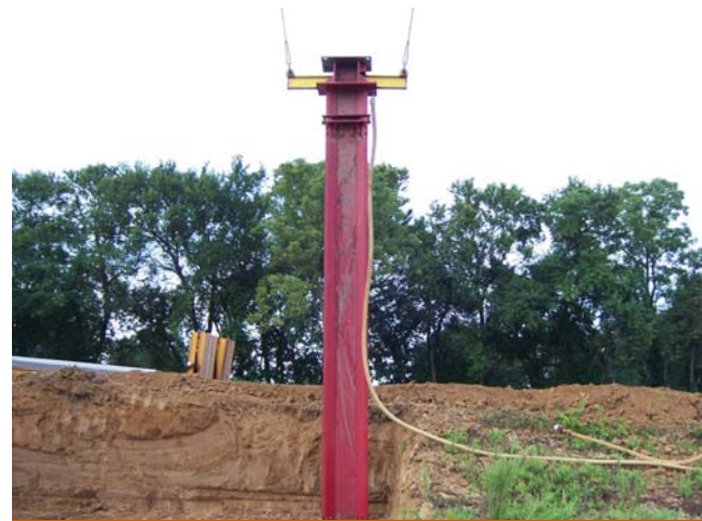
Typical steel mandrel encases HDPE sheet during installation.
