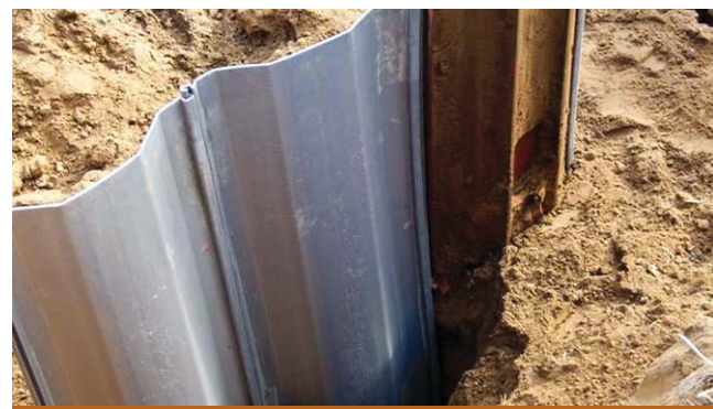
Close up of mandrel during installation.
