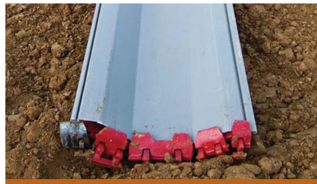
Toe clamps released after depth has been achieved.
