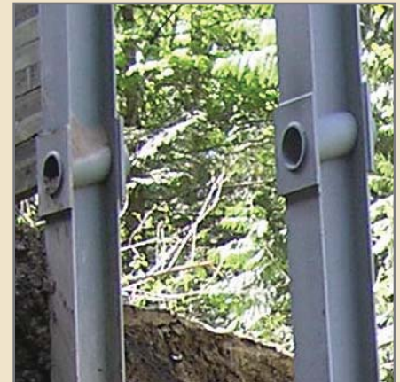
Schedule 40 black steel pipes with 9 5/8 inches x 7/16 inch pipe pockets
