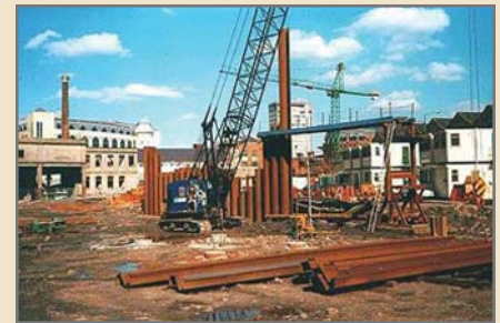
Phase 1: Sheet pile installation
