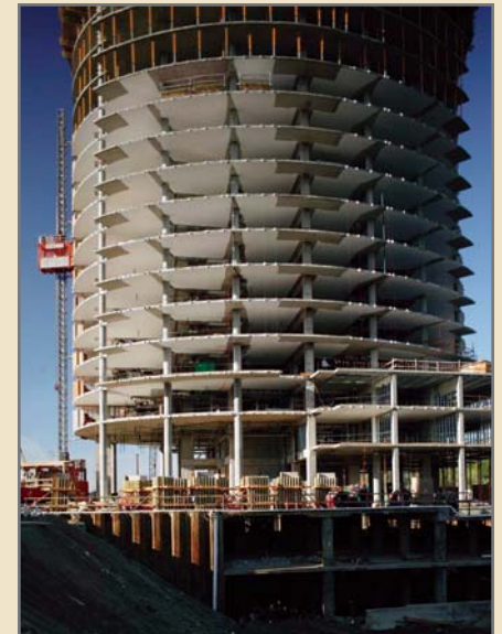
Concurrent above and below grade construction
