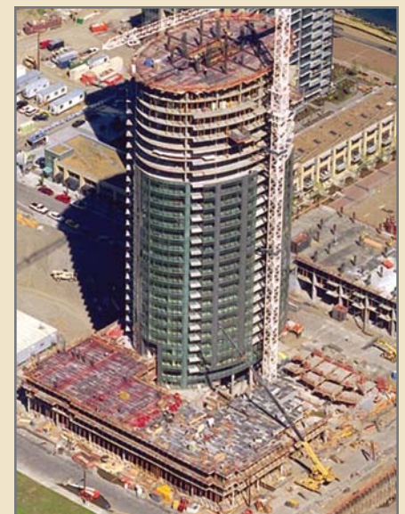
Aerial view of construction progress
