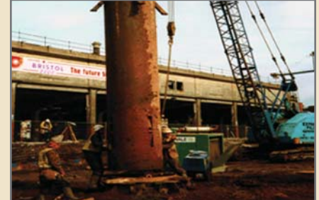
Concurrent: Pile Foundation Installation
