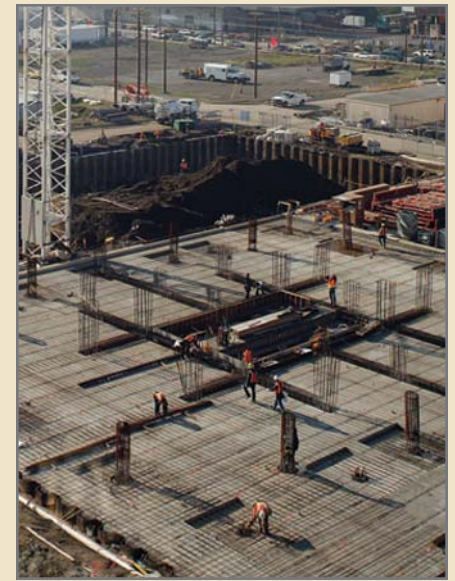
Site footprint of early foundation construction
