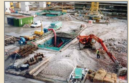
Access for below grade excavation
