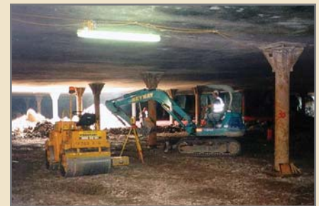
Phase 3: Below grade excavation
