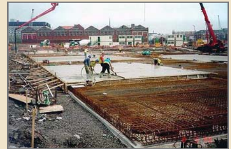
Phase 2: Base slab construction
