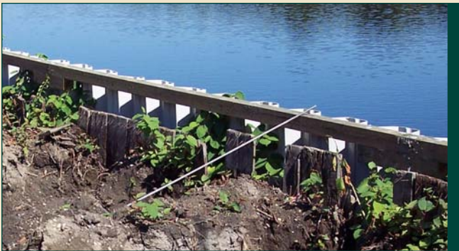
Installing anchored walls requires excavation 10'-20' behind the wall; homeowners love the cantilever option because it creates less disturbance to their property.
