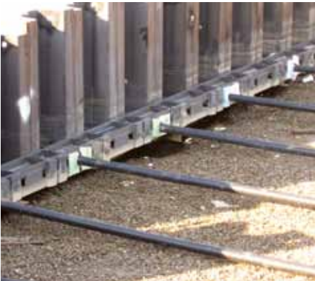
Double Corrosion Protection (DCP) Tie Rods
