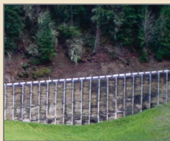
Completed ground stabilization wall
