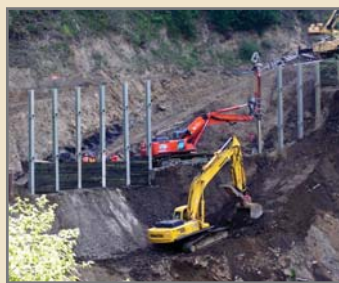
Construction of soldier pile wall
