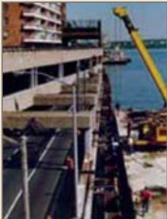
Sheet pile installation from marine barge on the East River
