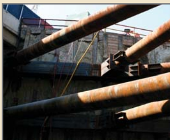
Spiralweld pipe struts support the internal section of wall
