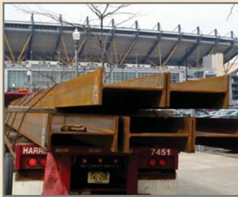
24-inch wide flange beams arriving at the site near Heinz Field
