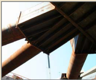
Fabricated pipe strut configuration
