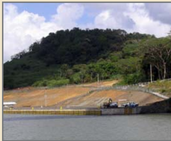
Completed tie up structure
