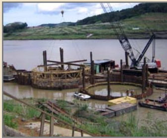
Template construction for cellular coffer dam
