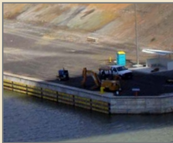
Final phase of dock construction
