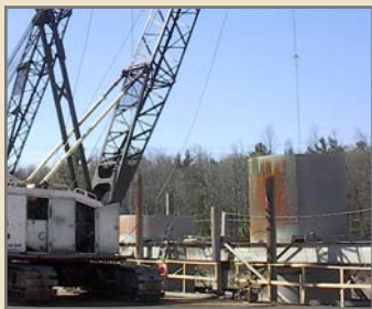
Caissons placed in rigid template frame.
