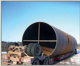
Steel casing being delivered to site.
