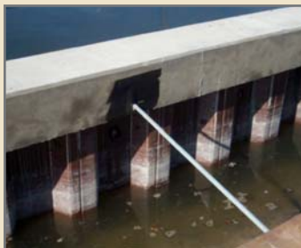
Concrete structural cap and tie-back nearing wall construction completion
