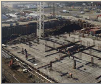
Site footprint allowed for innovative hybrid top down construction method
