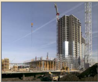
Foundation work is off the critical path at the earliest stage
